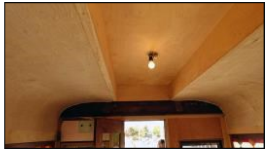
New curved roof in Lounge Area
