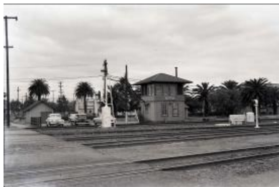
Photo 3 - Tower in 1954 from Brokaw Rd. Crossing, John Harder photo, Dave Hambleton collection
